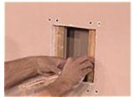
If you can't find drywall the correct thickness, glue shims to the braces and use slightly thinner drywall.
