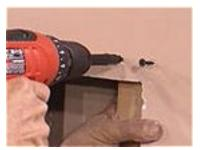
When you're working without a helper, start the screws to simplify attaching the braces. Pull the brace tightly toward yourself as you insert the screws.
